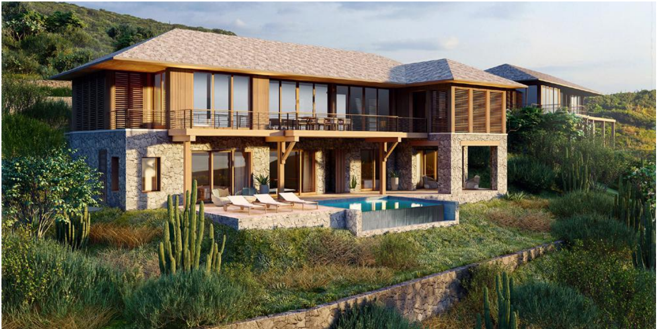
FIGURE 13: EXTERIOR WALLS UTILIZE A MIXTURE OF STONE AND WOOD TREATMENTS TO BLEND BUILDINGS INTO THE SITE.
