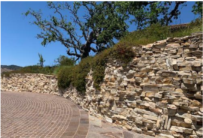
Examples of stone retaining walls utilizing regional dry-stack patterns.
